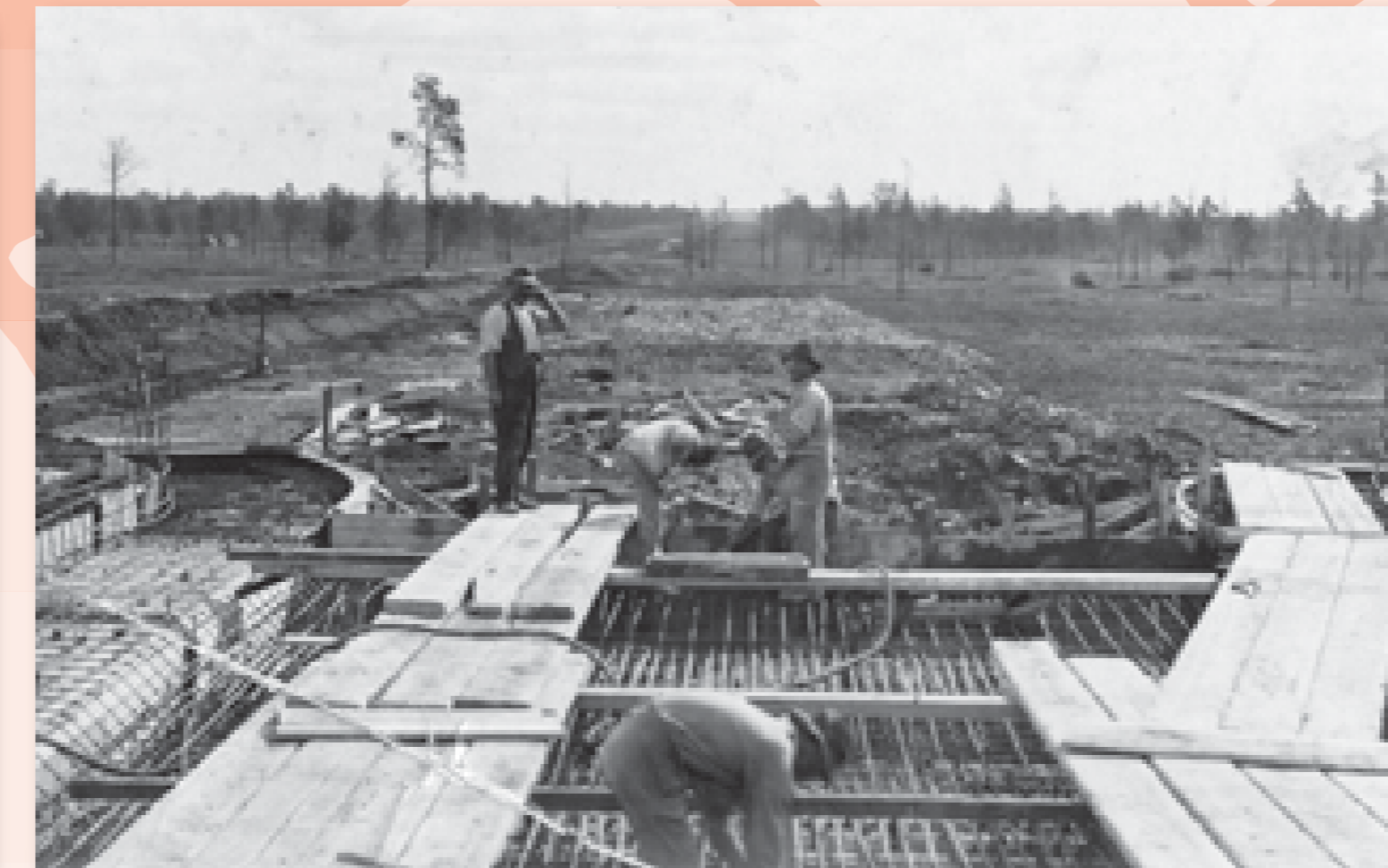
3. Foreman Nightingale inspects completed canal construction work (date unknown)
